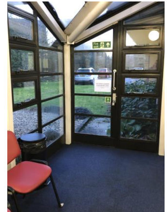
Unblocked fire exit
